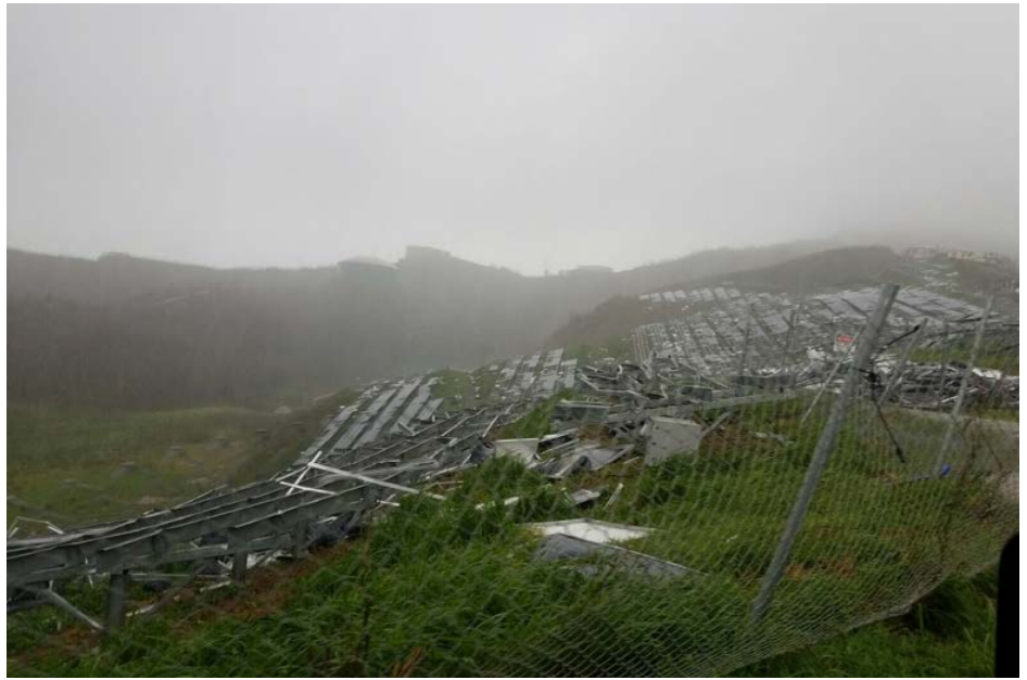
Damaged USVI 1 solar field on St. Thomas; Source: Kelsey Nowakowski
